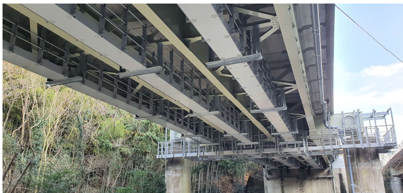
Yamanaka Viaduct, Kanmon Expressway
