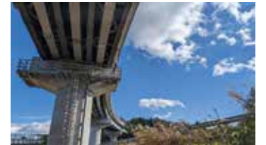
An FRP inspection passage makes bridge maintenance safer and easier (Iwate Prefecture)
