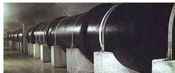
A ductile iron pipe laid in a tunnel
